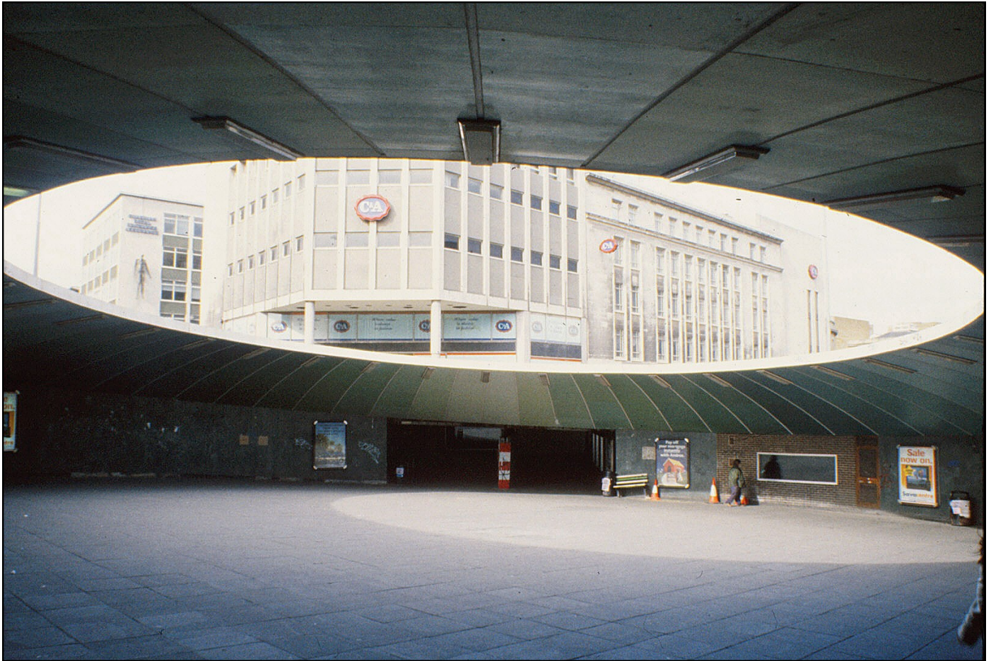
Castle Square, looking north-east (1993)
