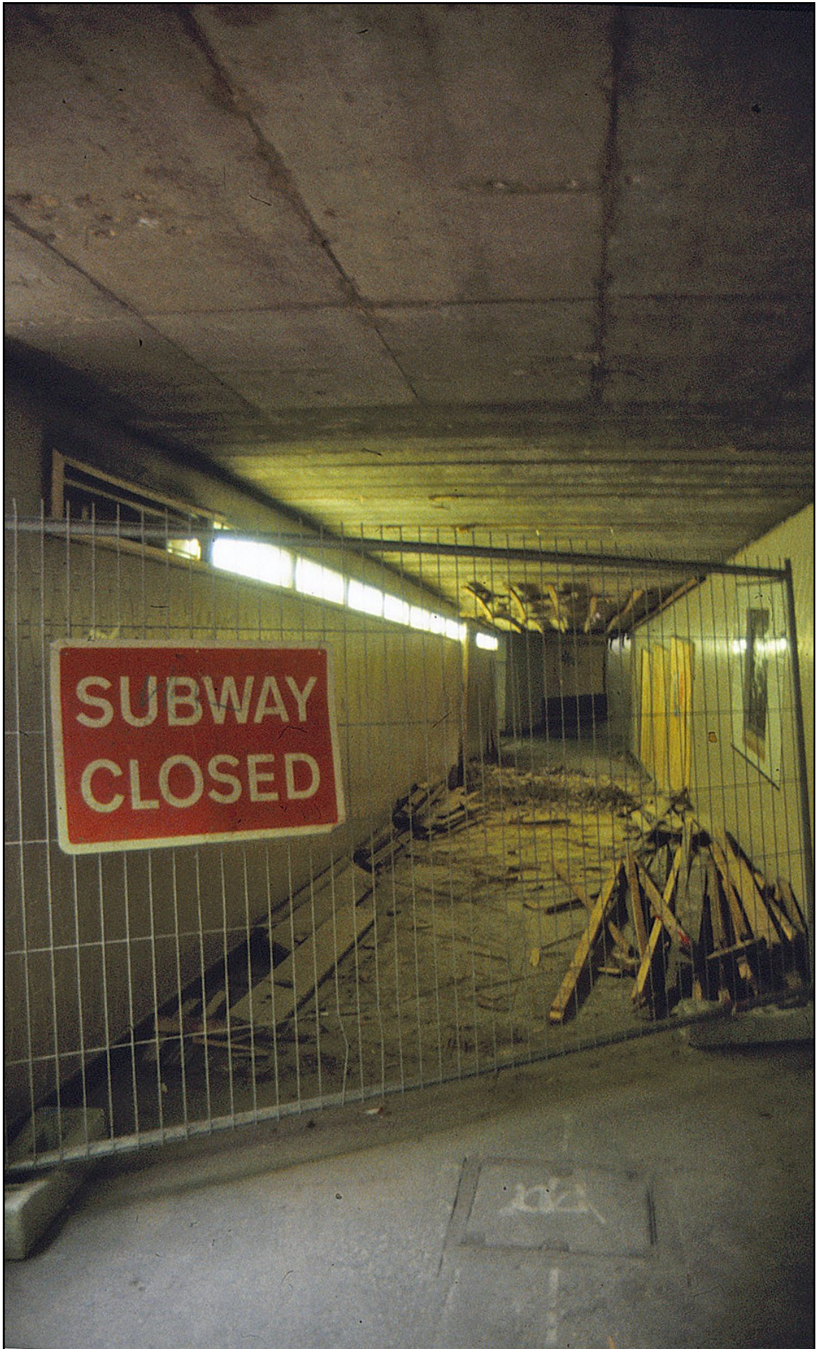
Castle Square – demolition (1994)
