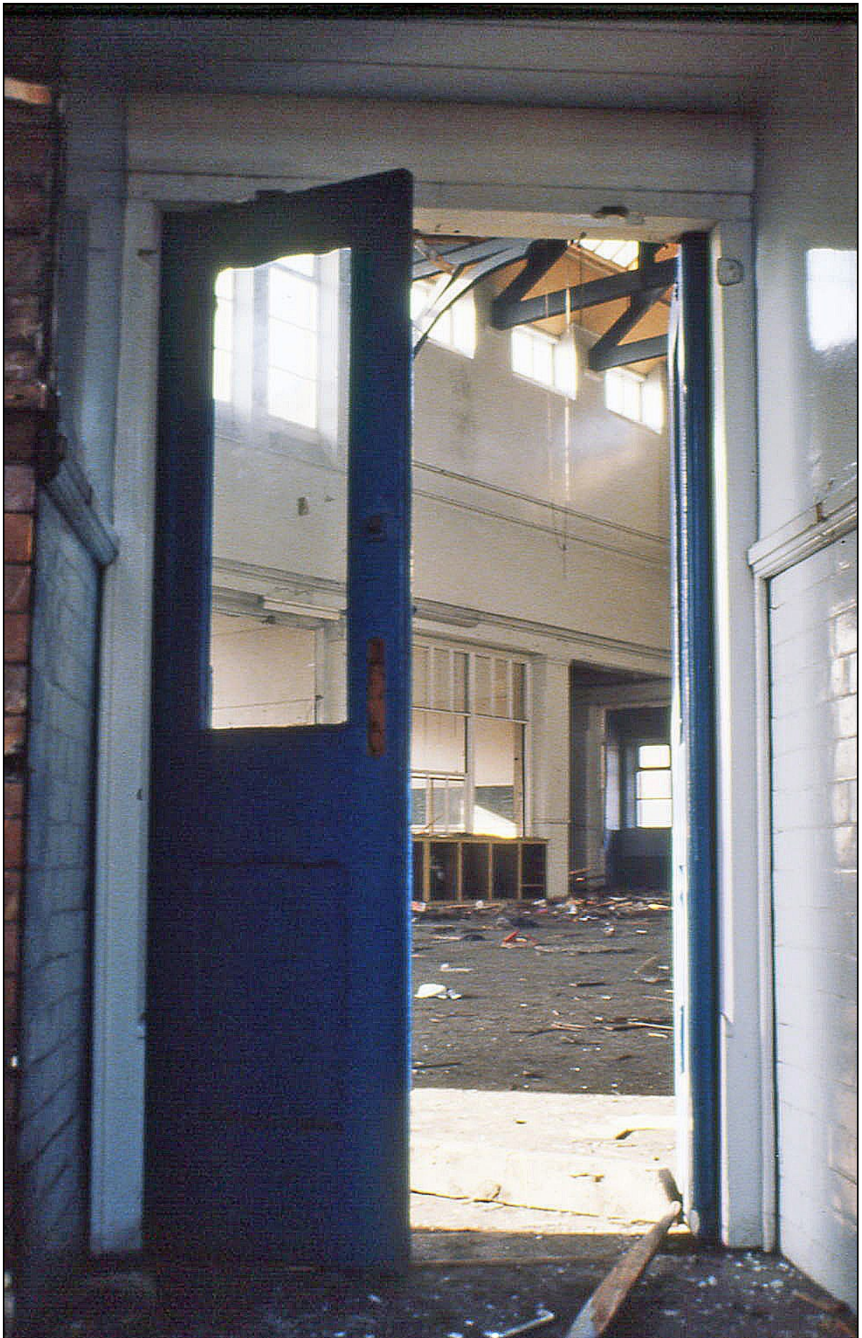
Huntsman's Gardens Schools assembly hall – demolition (1980)
